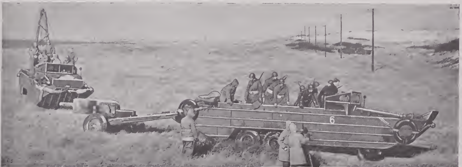
FIGURE 96. 105-mm howitzer unloaded from one DUKW with aid of A-frame on another is hauled into battery position.
